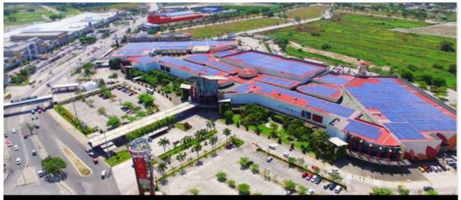
Commissioned in May of this year, Robinsons Starmills' 2.88 Megawatt peak solar rooftop is currently the largest solar powered shopping mall in the world. The system is expected to offset 2,480 tons of CO2 emissions on its first full year of operation.
